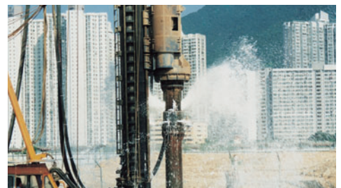
Foundation Foundational construction of buildings and bridges up to 32"(ø800) of casing diameter.
